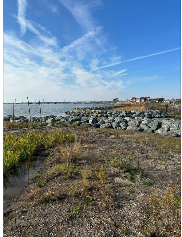
Natural and nature-based features were utilized in the installation of a living shoreline in Patchogue, NY. Photo: NYSG/K. Fallon
