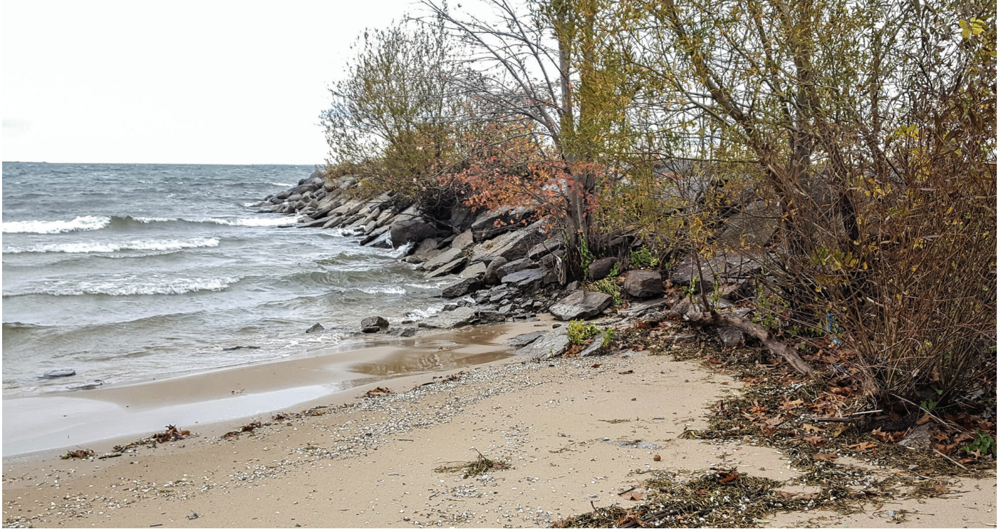
Small rubble mound groin with vegetation, Westcott Beach State Park. Photo by Roy Widrig, New York Sea Grant.
