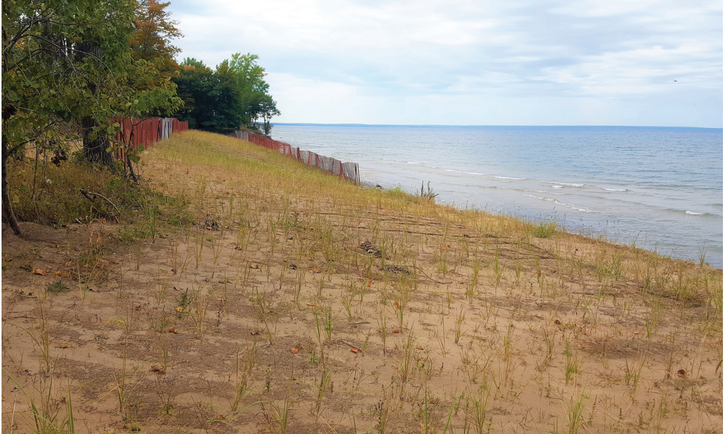
Ongoing dune revegetation and sand fencing placed at Sandy Island Beach State Park. Photo by Roy Widrig, New York Sea Grant.
